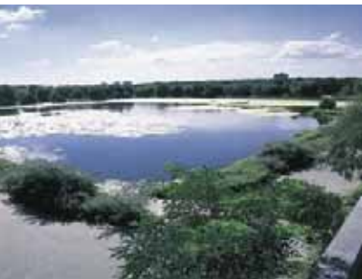
Infiltrationsbecken in Berlin Recharge Pond in Berlin
