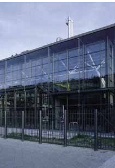
Abwasserpumpwerk Sewage pump station
