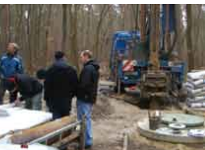
Messstellenbau Construction of an observation well
