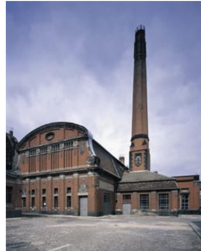
Abwasserpumpwerk | Sewage pump station
