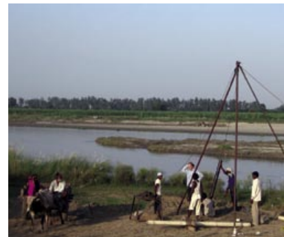
MAR-Systemanlage in Palla Field Site | MAR systems installation at Palla Field Site
